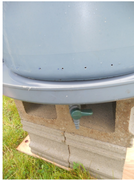
Figure 3.2: Drainage holes and collecting tray
