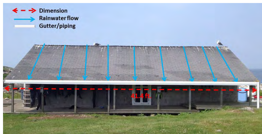
Figure 7: Front view of the Dive Shack, with a vertical 550 gallon HDPE cistern for catchment and a gutter system.
