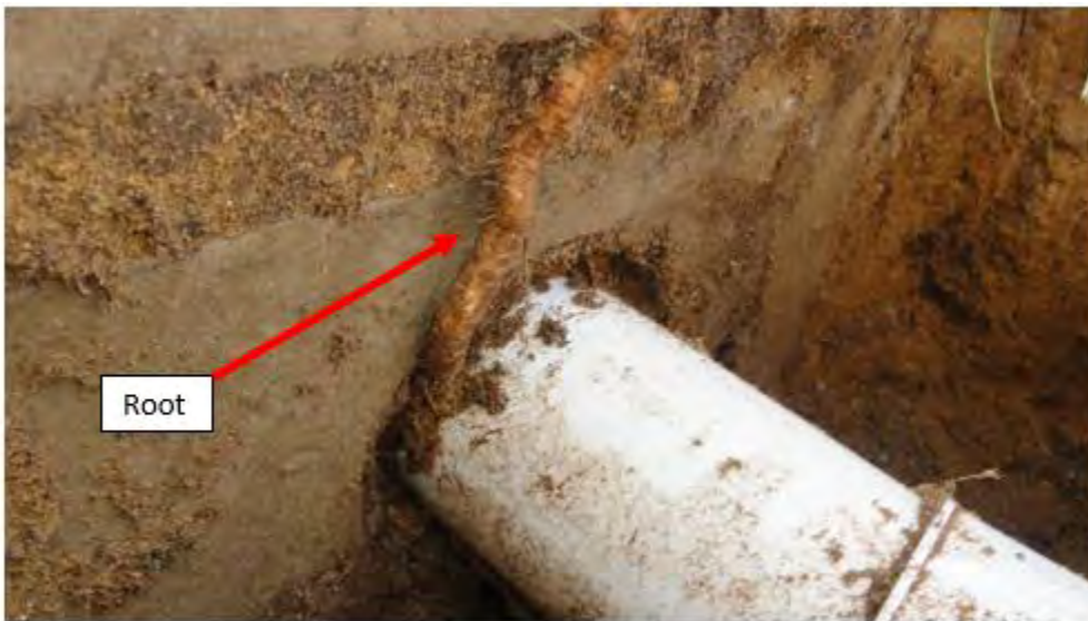
Figure 7.6 - Root entering the outlet of FRICKle FILTER™
