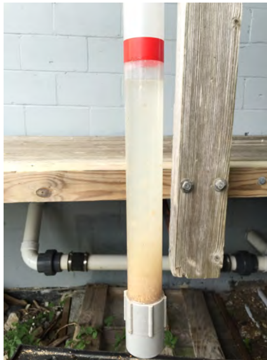
Figure 31: Grease Interceptor Coring Sample of Effluent
