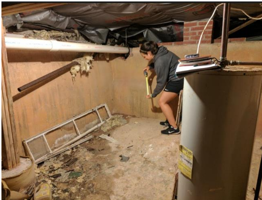
Figure 13. Picture of the existing cistern in the basement of Founder’s Hall
