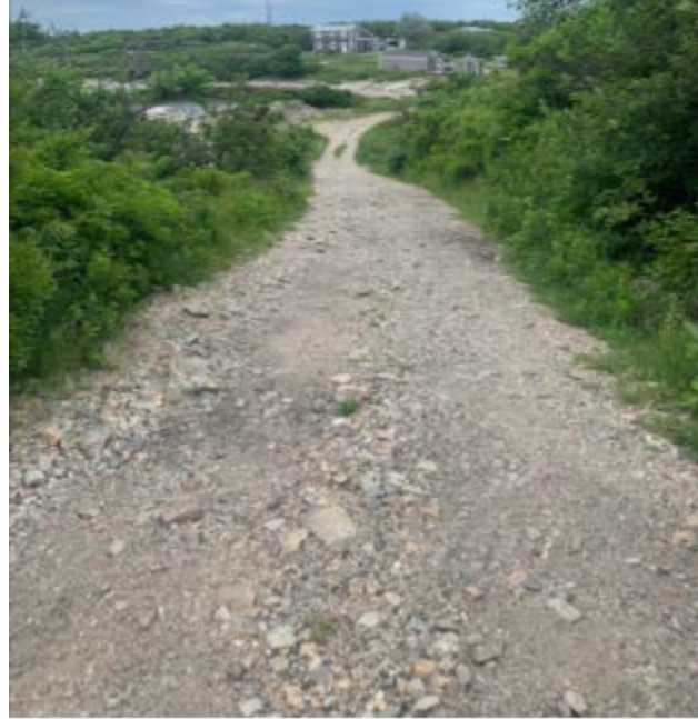
Figure 4.9: Below culvert on coastal slope on western side of island, 6/16/2022
