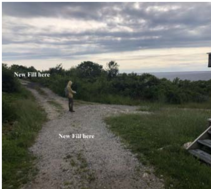
Figure 4.14: Fill on Site 2, 6/16/2022
