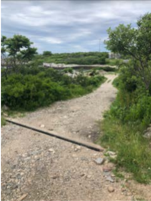
Figure 4.8: Culvert on coastal slope on the western side of the island 6/16/2022
