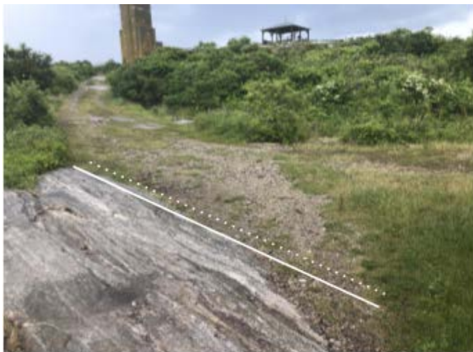
Figure 4.26: Ledge enhanced as natural level spreader; dig in front to create more of a ledge, implement riprap on side to help drainage into surrounding vegetation.
